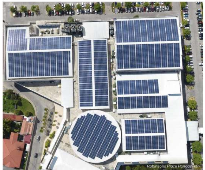
Robinsons Place Pangasinan
